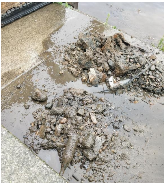
Figure 14: Photos from Sampling (Location 2)
