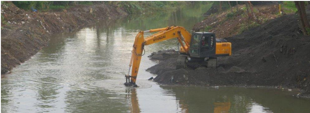
Figure 4: Dredging by excavator from the river channel
