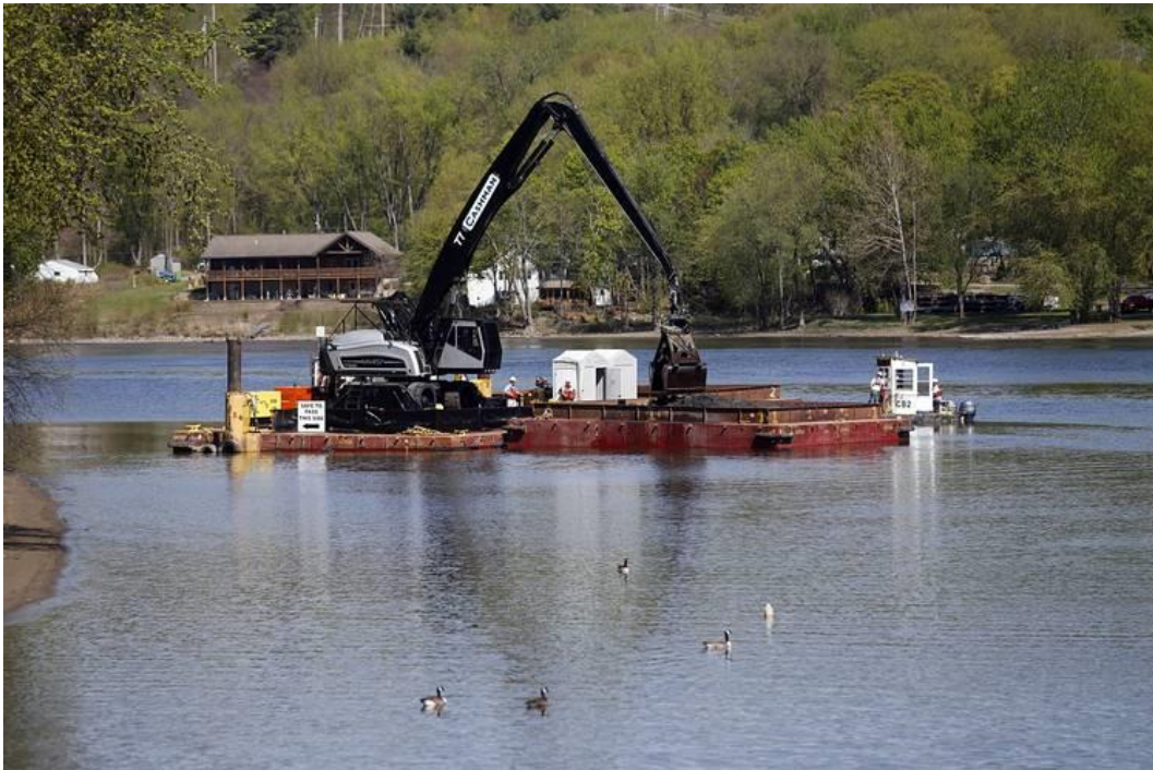
Figure 5: Example of a barge equipped with excavator
